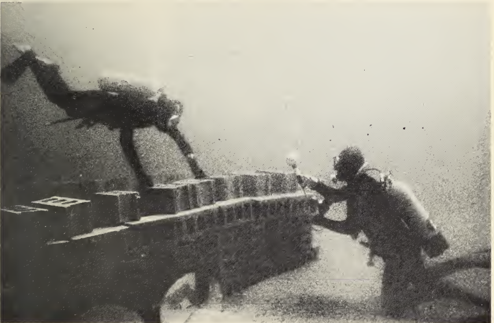
An artificial reef of concrete blocks was built near Sublimnos on a barren plain of sand. It attracted a great many animals, particularly at night.
